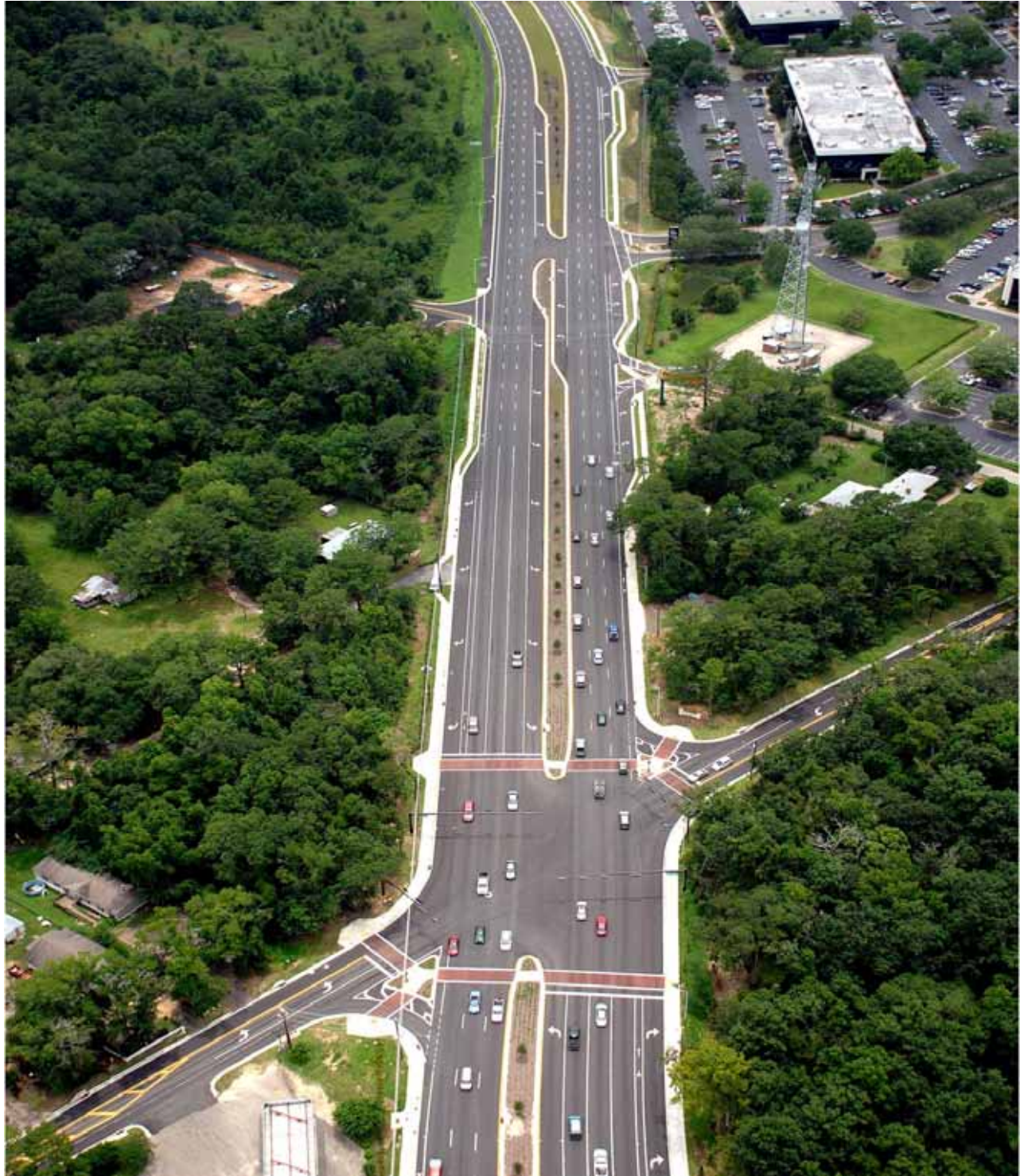
CCSE – The Old St. Augustine Road Intersection Looking South
