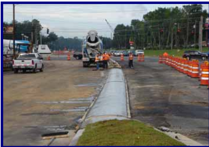
Placing Class I Concrete for Traffic Separator Tennessee St.
