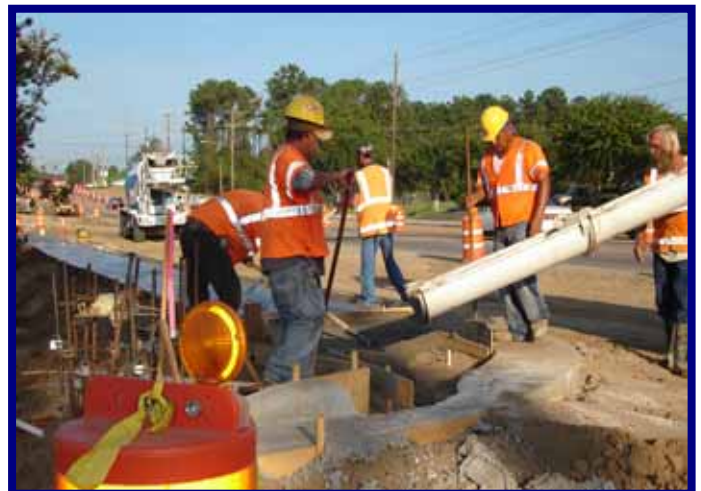
Placing Class I Concrete for sidewalk on Tharpe St.
