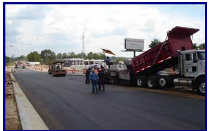
Placing Asphalt Base on Tharpe Street
