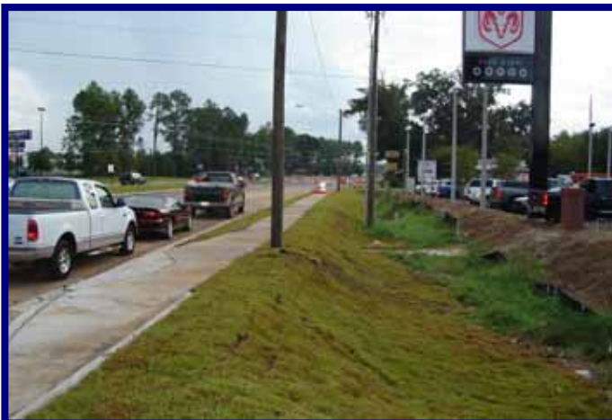
Placing Sod right of right roadway Tennessee St.
