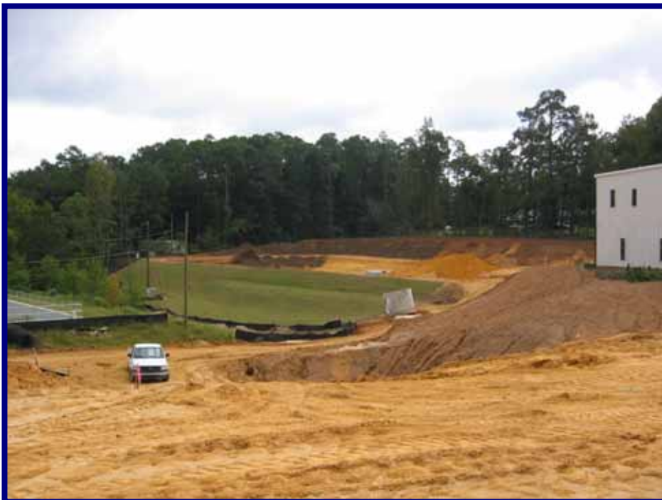
Capital Circle Southeast Segment Two – Pond 11
