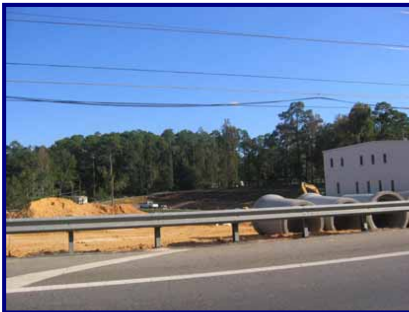
Construction on Pond #11 Segment 4
