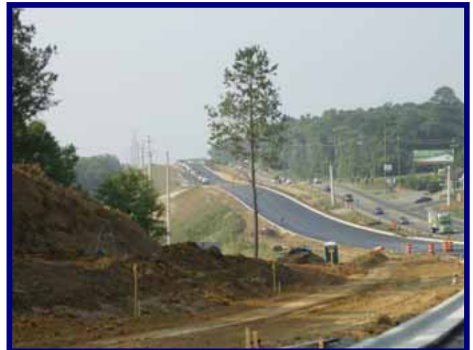
Segment 3 – Paving Operation
