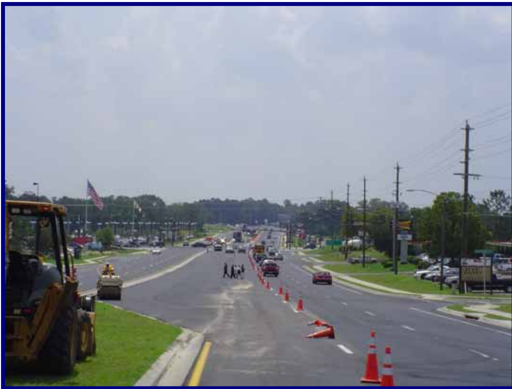
CCNW Placing Friction-Course Asphalt at CCNW / Tennessee Street Intersection
