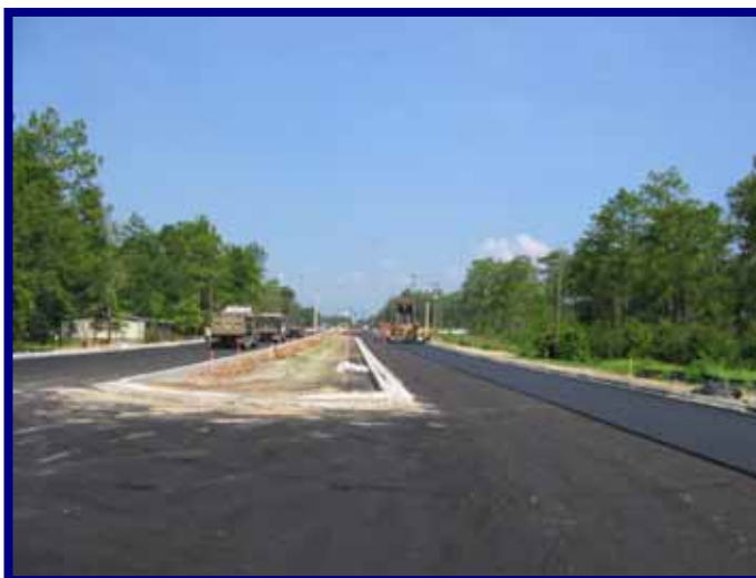
Paving Tram Road East of CCSE
