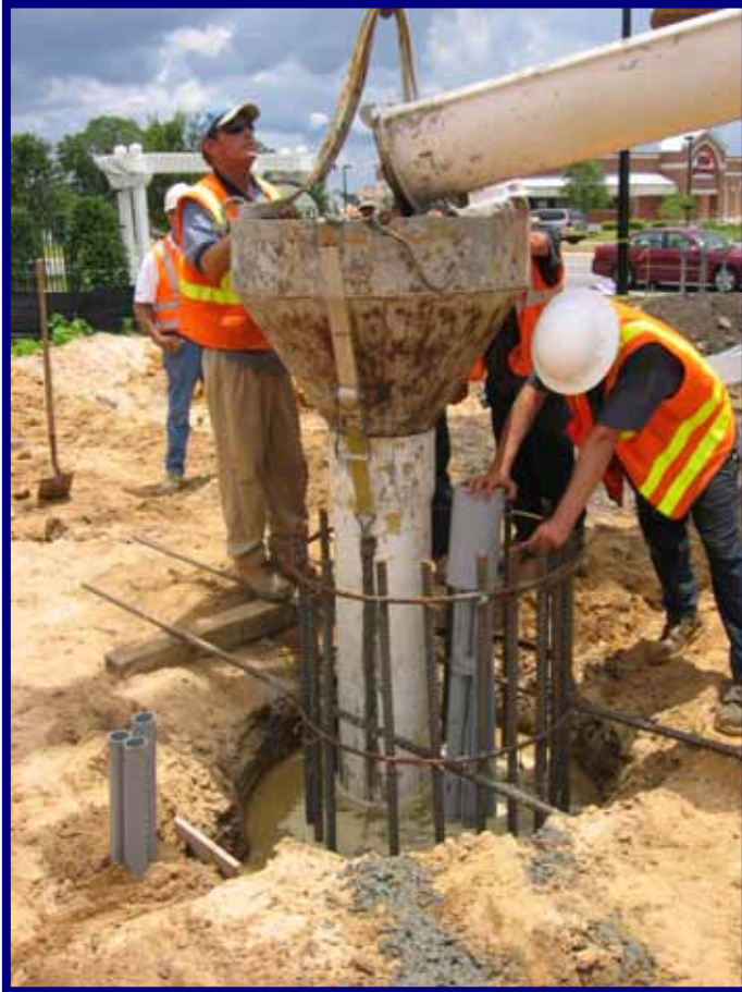
Putting in Mast Arm Base
