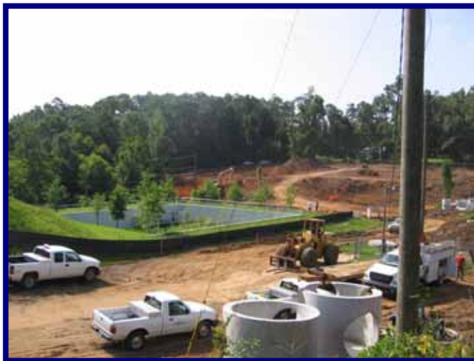
Pond 11 Construction in Segment 4
