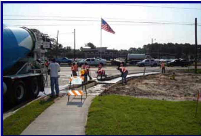
August 7 2006 – Placing Sidewalk
