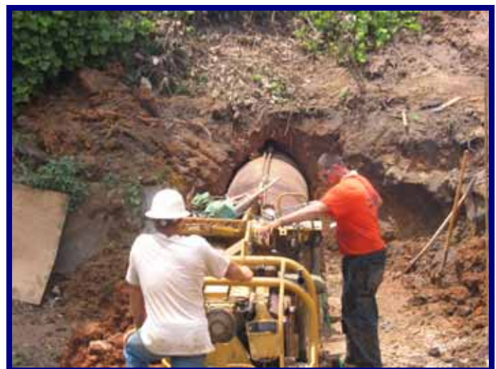
36" Pipe at Ravine in Segment 4
