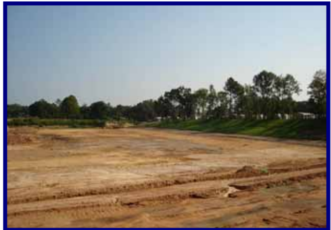
August 7, 2006 – Pond 1 Excavation.
