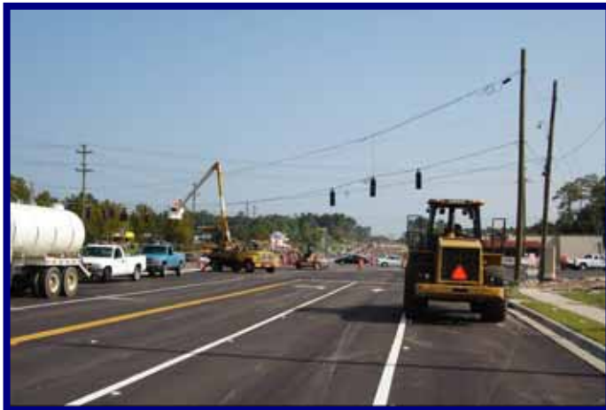
Installing Temporary Signals
