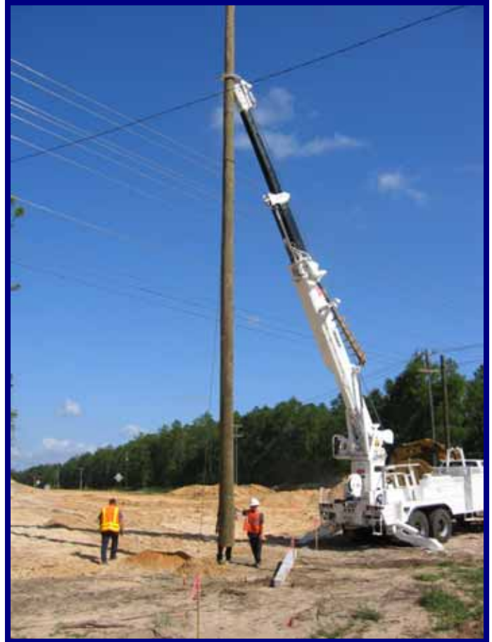
Placing Mast Arm
