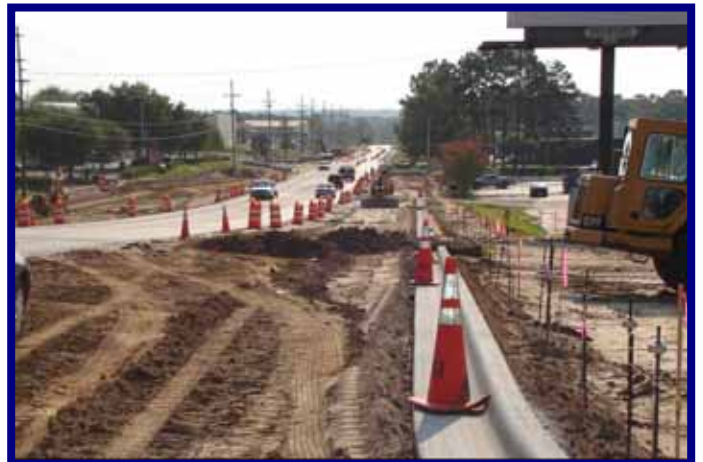
Placement of Type F curb & Gutter – E. Tharpe St.
