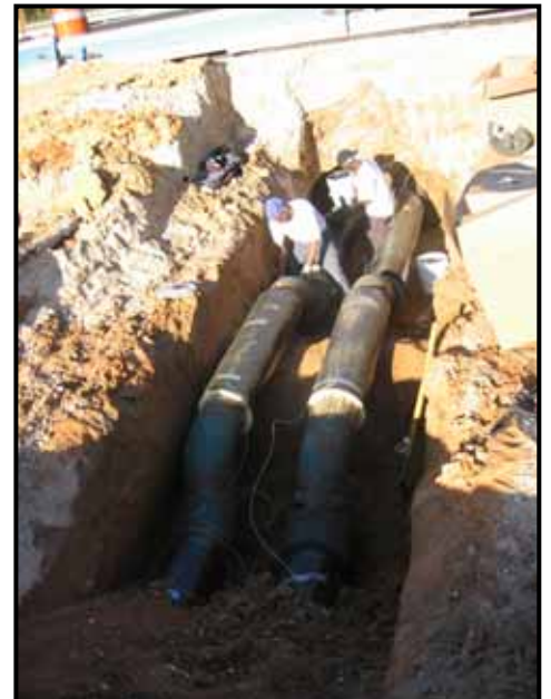
Installation of chilled water lines.
