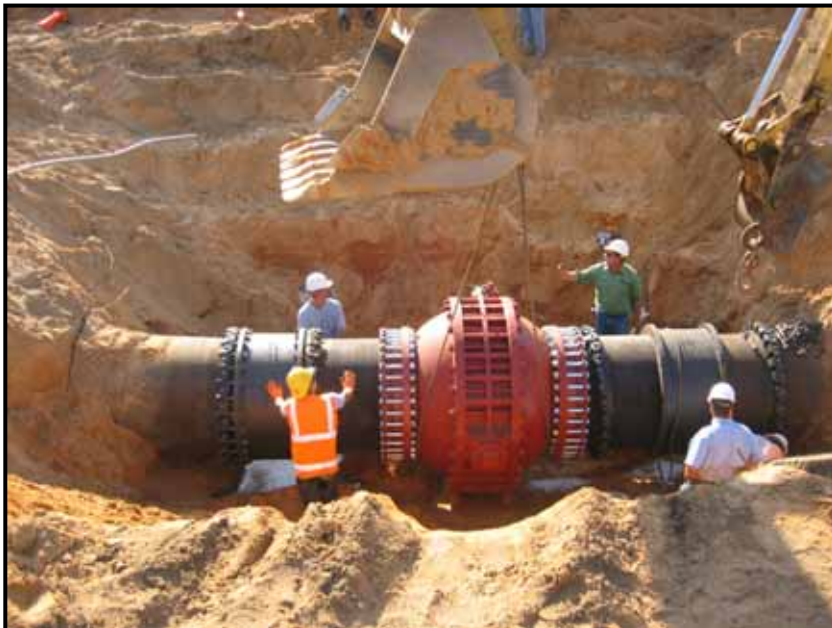
Installation of valve for 30" Sanitary Bypass.
